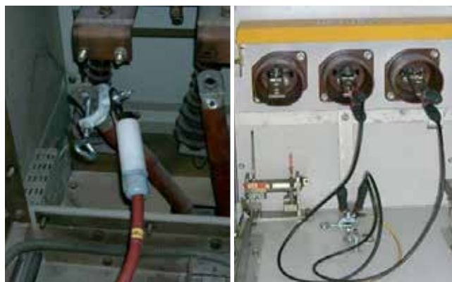
➤ single phased connection, not involved phases grounded
