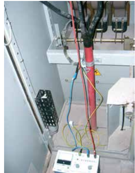
➤ galvanic connection of audio frequency generator TG
