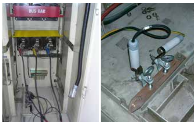
➤ 3 phased connection, common grounding point of safety earth and operation earth clamps
