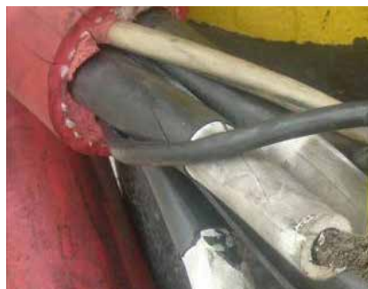
➤ 3-core EPR, incl. dataline, radial type
