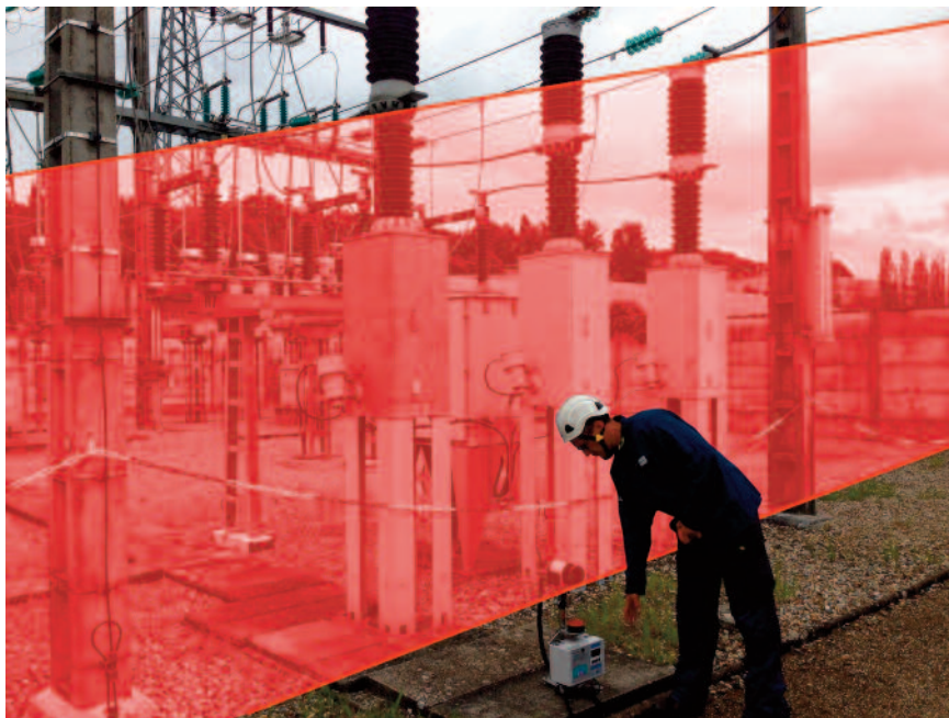
Maintenance operations in a high voltage ub-station
